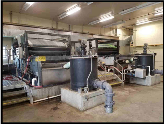
Left: Existing Belt Filter Press from 1988 is becoming increasingly more of a cost burden to maintain.
