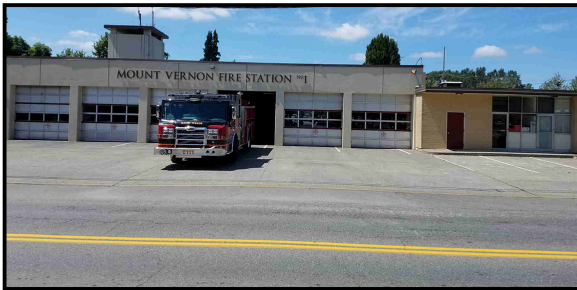
Apparatus bays leave little room on either side of trucks to fit in and out doors. Ladder truck cannot fit in this station. Poor lighting inside results in dark interior when backing up.
